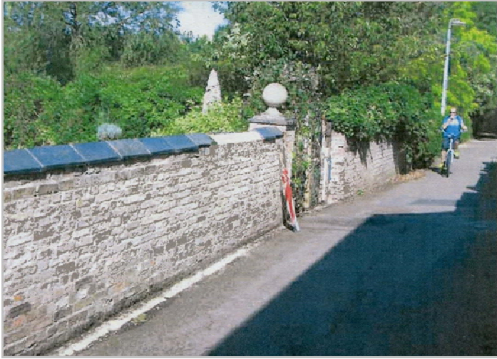
Wall prior to demolition
